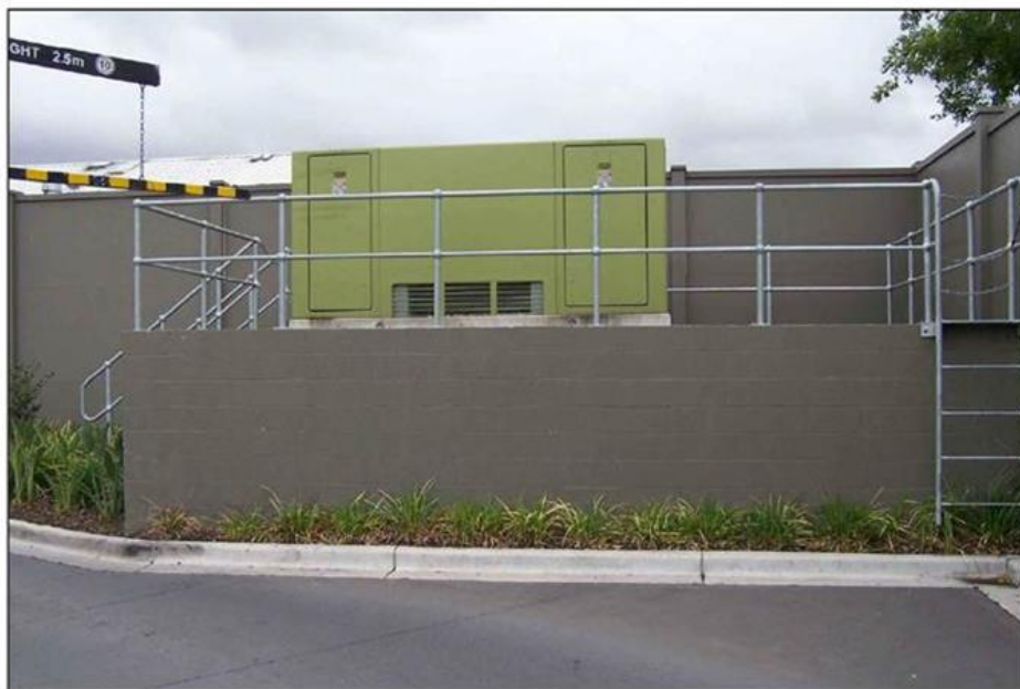
Figure 51 - Example substation raised above 1:100 flood level
